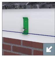
Fix fascia brackets with Alutec 32mm x No. 10 roundhead screws, code SC201 or Alutec 15mm x No. 10 countersunk screw, code SC203 if fixing to Alutec aluminium composite fascia. Insert screw into lower slot and adjust to the string line.
