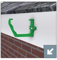
Fix fascia brackets with Alutec 32mm x No. 10 roundhead screws, code SC201 or Alutec 15mm x No. 10 countersunk screw, code SC203 if fixing to Alutec aluminium composite fascia. Drilling pilot holes first is recommended.
