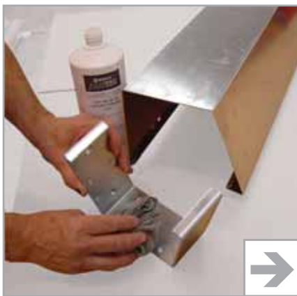
1. Clean all jointing surfaces with clean cloth and solvent cleaner, SC108.
